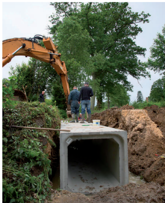
Installation of a rigid-frame bridge on an affluent of the Rouvre.
