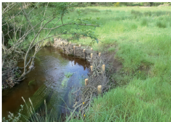
Restoration of banks damaged through cattle watering (left) by the installation of willow fascines (right) on the Bonne Chère.
