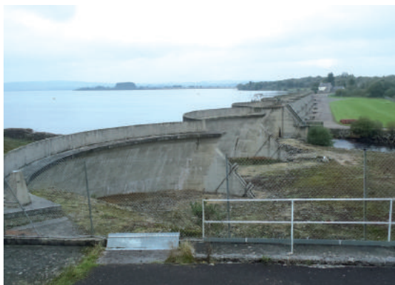
The Nestavel Dam on the main stem of the Elez River.
