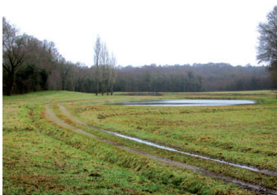
Lagoons at the Malguénac wastewater treatment plant in the Bonne Chère watershed.
