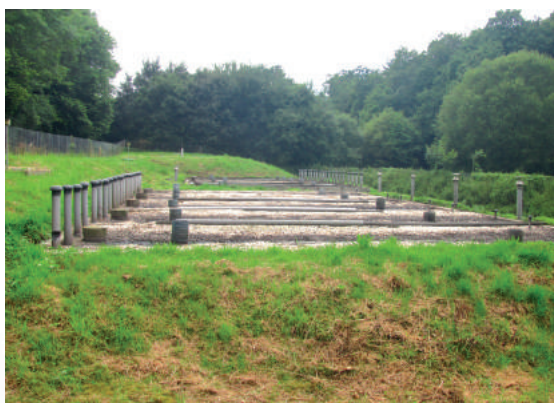
The Carneille wastewater treatment plant in the Rowre watershed.
